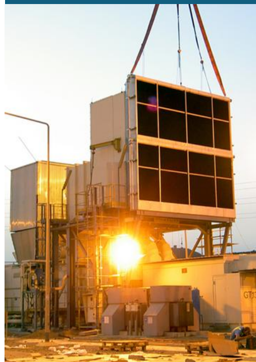
Installation of Munters evaporative air coolers
